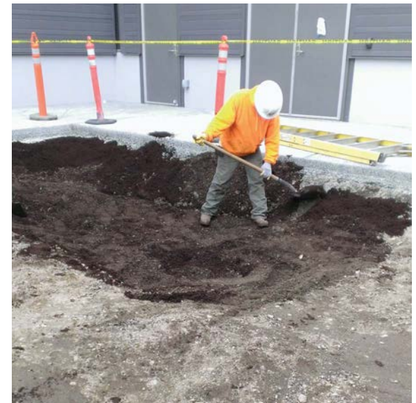
Example soil preparation: subgrade preparation
